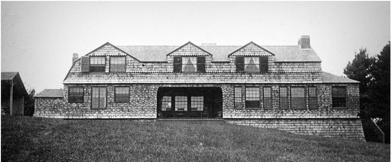
Percy Browne House, Marion, Massachusetts, c. 1902. H. H. Richardson, architect. Courtesy Sippican Historical Society.
