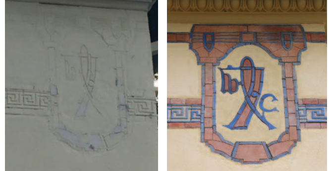
L to r: The exterior tilework was obscured by plaster and paint. The vibrant tilework medallion is revealed; the ensign of William Caxton, 15 th century British printer. Courtesy Northwest Vernacular Historic Preservation.
