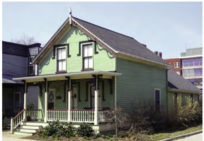
The Gothic Revival house in its new location after moving and a complete restoration by the Cleveland Restoration Society.
