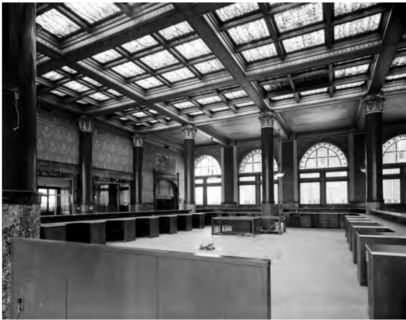
Society for Savings, interior, Banking Room. Burnham and Root, architects. William Pretzman, interior designer, 1887-1890. Historic American Buildings Survey.
