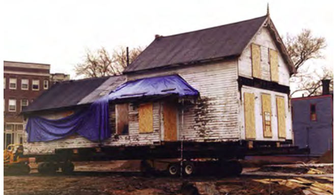
The house on its way around the corner.
