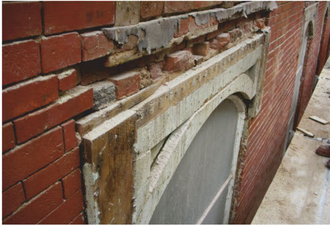
(L to R): Window before restoration, after removal of the Formstone. Window after completed restoration.
