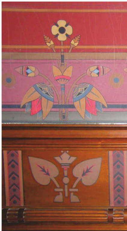
Beginning on the walnut dado border, separated from the recessed paneling by a carved bundle of reeds, is a painted foliate motif of a plant with spade-shaped leaves
