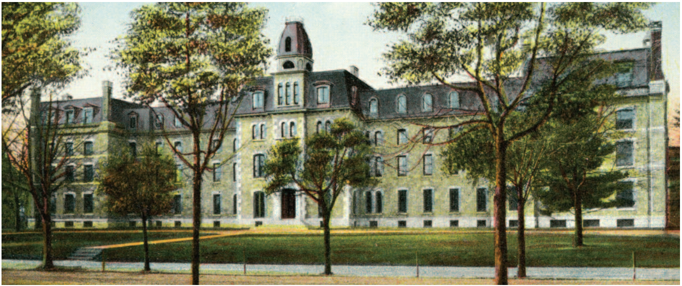
The Normal School Building, c. 1871. West Chester, Pennsylvania. Addison Hutton (1834-1916), architect. This building was the first of seven constructed with serpentine stone on the school's campus. Author's collection.
