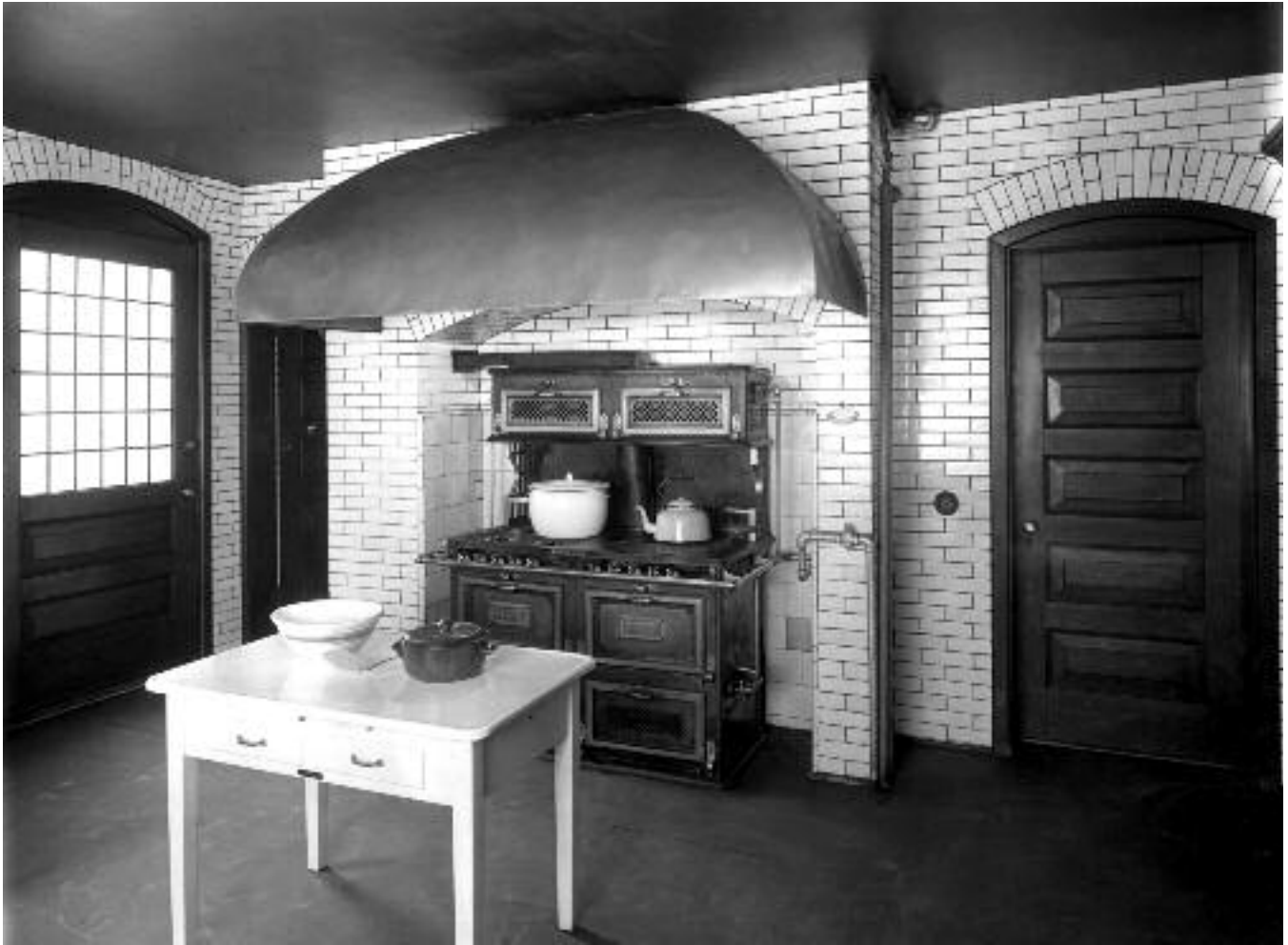
The Glessner House kitchen, photographed in 1923 by Kaufmann & Fabry Co. The door to the right of the stove leads to the servants hall. To the left is an exterior door leading to the service courtyard. Partly visible to the left of the stove is a door leading to a storage pantry and a walk-in cold room. The kitchen's durable glazed brick walls are visible, although its original encaustic tile floor had been covered over by the time this photograph was taken. Courtesy Glessner House.
