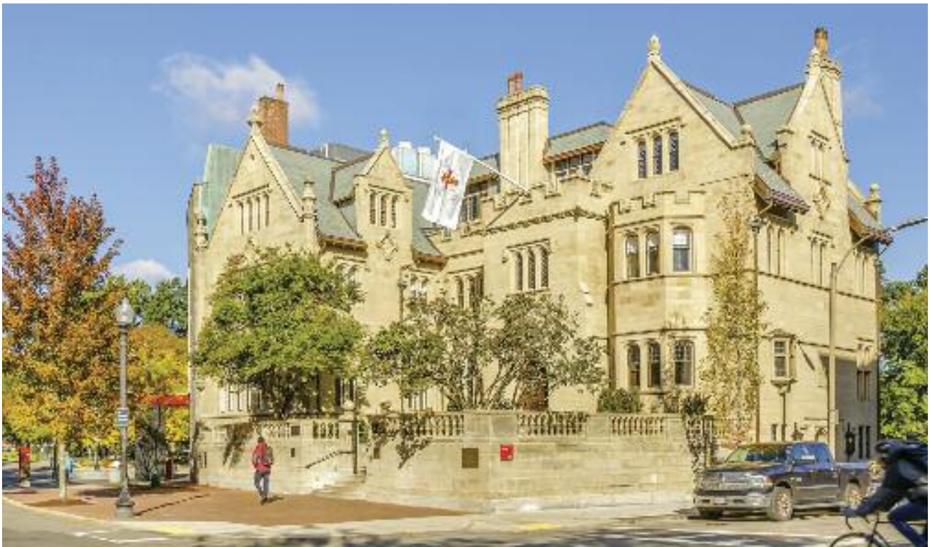
Exterior of the completed Dahod Family Alumni Center shows the repaired and cleaned stonework and roof details. Photo by Raj Das Photography.
