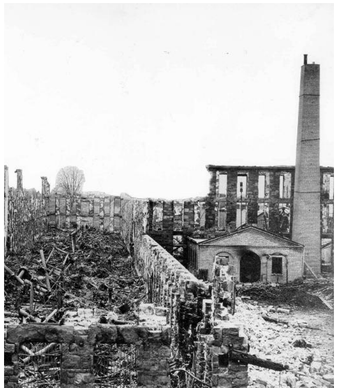
The original Colt Fire Arms Manufacturing Company, after it was destroyed by fire, February 1864. Courtesy Connecticut State Library.
