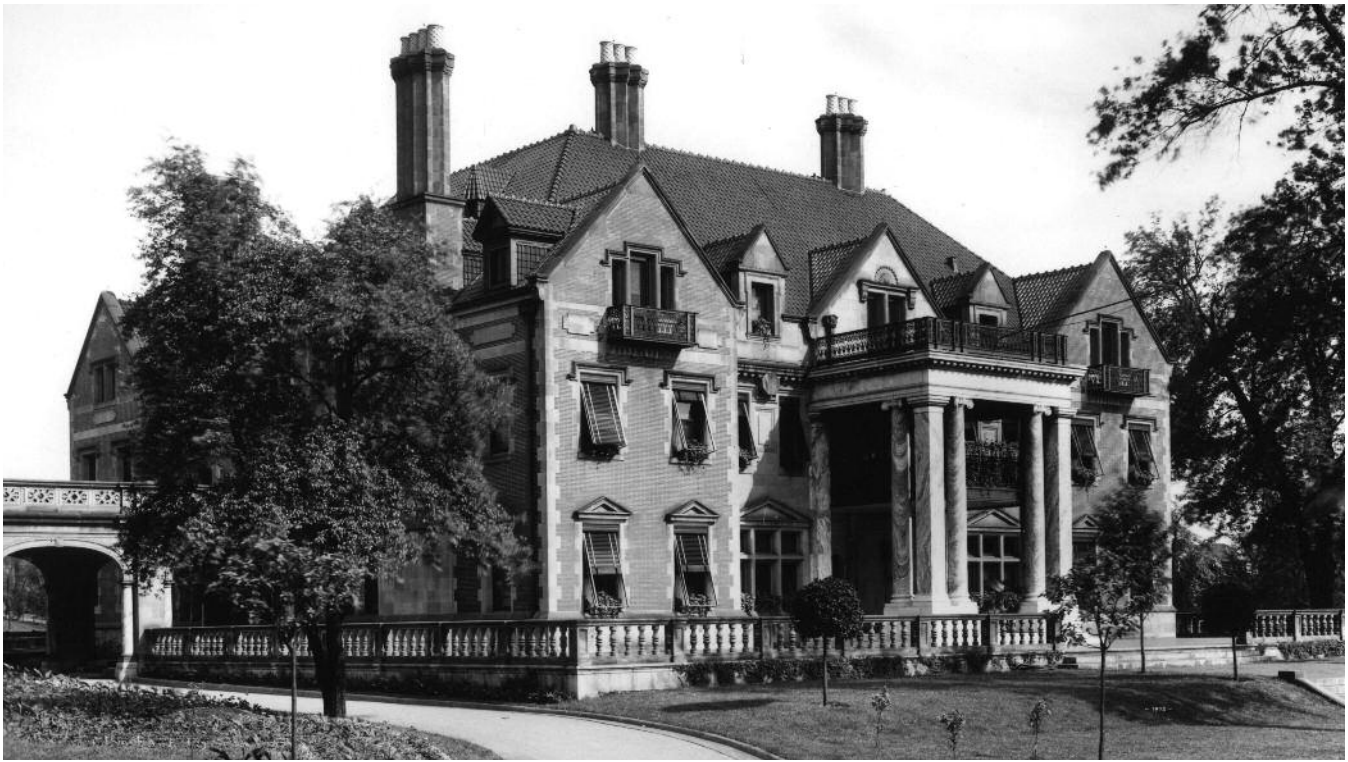
Rowanlea, the Peacock residence, Pittsburgh, Pennsylvania, c. 1904. Alden & Harlow, architects. R. W. Johnston, photographer.
