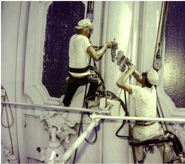
L to R: Removal of paint inside the dome, c. 1960. Interstitial space of the dome after painting and final cleaning, 2016. Cleaned section of the external coffered dome, 2016. Photos by Chuck Badal. Courtesy of the Architect of the Capitol.
