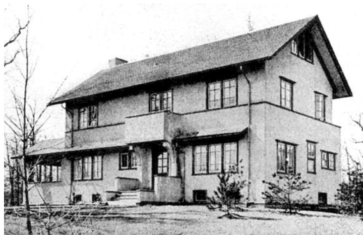
The William E. Davis house, 1906, Winnetka, Illinois, which Spencer merely identified as "a typical simple house with rough cast exterior." House Beautiful , September 1908. Robert C. Spencer, Jr., architect.
