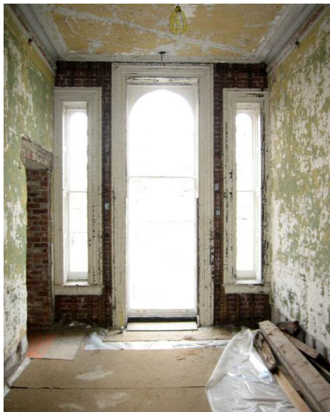
Top to bottom: Interior conditions before construction, looking north along the central corridor. Looking west through the original tripartite wood windows and surrounds with integral shutters. Courtesy Gluckman Tang.
