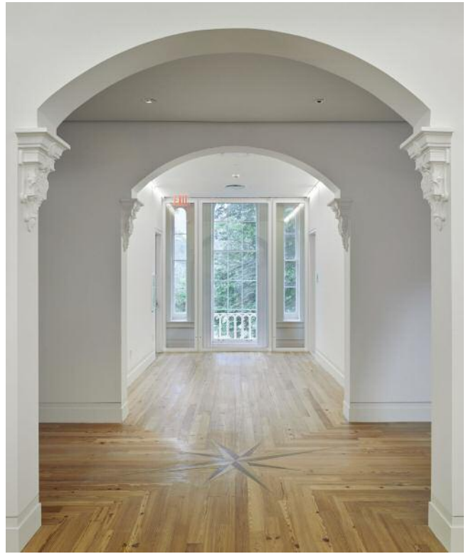
L to R: Looking east toward the A/B Hyphen. Original corbels and archways were replicated and adjacent cast-iron staircase restored. Courtesy Gluckman Tang. East view after restoration and renovation. Photo by Bruce Damonte.
