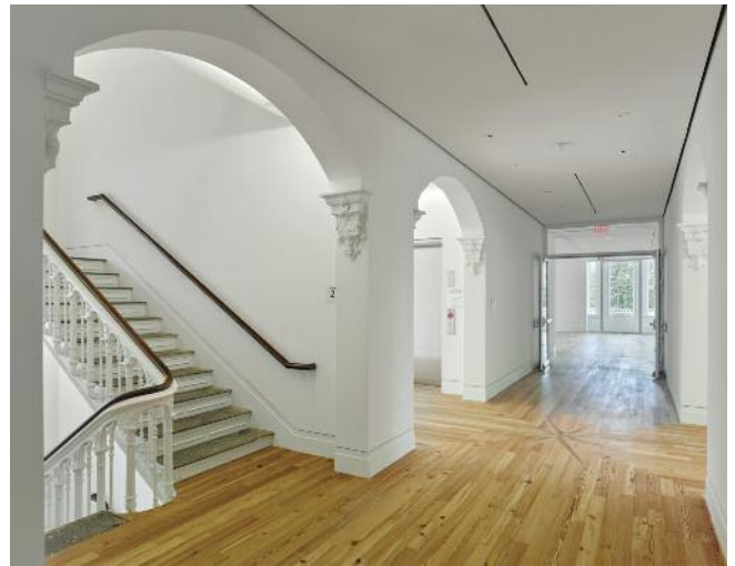
Above: Exterior of the restored Building A and A/B Hyphen. Below: Interior hallway with restored cast-iron staircase. Photos by Bruce Damonte.
