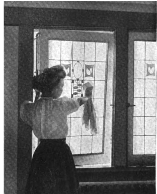
L to R: Exterior of Robert C. Spencer, Jr.’s home, River Forest, Illinois, illustrating the use of casement windows. Mrs. R. C. Spencer, Jr., demonstrating the cleaning of a casement window from the interior of the home. Spencer praised casements as “a great comfort after a hot summer’s day.” House Beautiful , July 1908.
