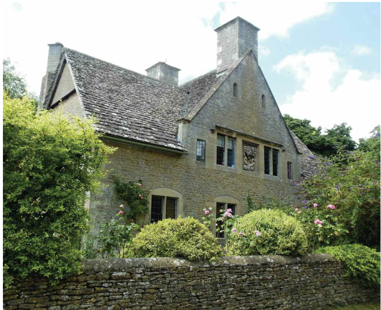
Kelmscott, Memorial Cottages. Designed by Philip Webb, 1899. Built 1902-1903. Photo by author. Courtesy of the National Trust.
