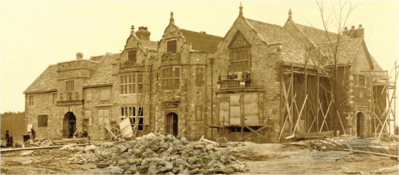
Virginia House, Richmond c. 1927. Note the forms of Warwick Priory's gables, reconfigured at center. Courtesy Virginia Historical Society.
