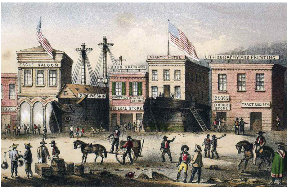
San Francisco, c. 1850. Another contributing factor to the success of Hutchings's publications was the location of his firm in the heart of San Francisco's business and publishing district.
